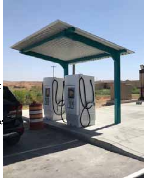
Photo (Above): Overton Power District's chargers installed in Mesquite, NV. (source: OPD).
