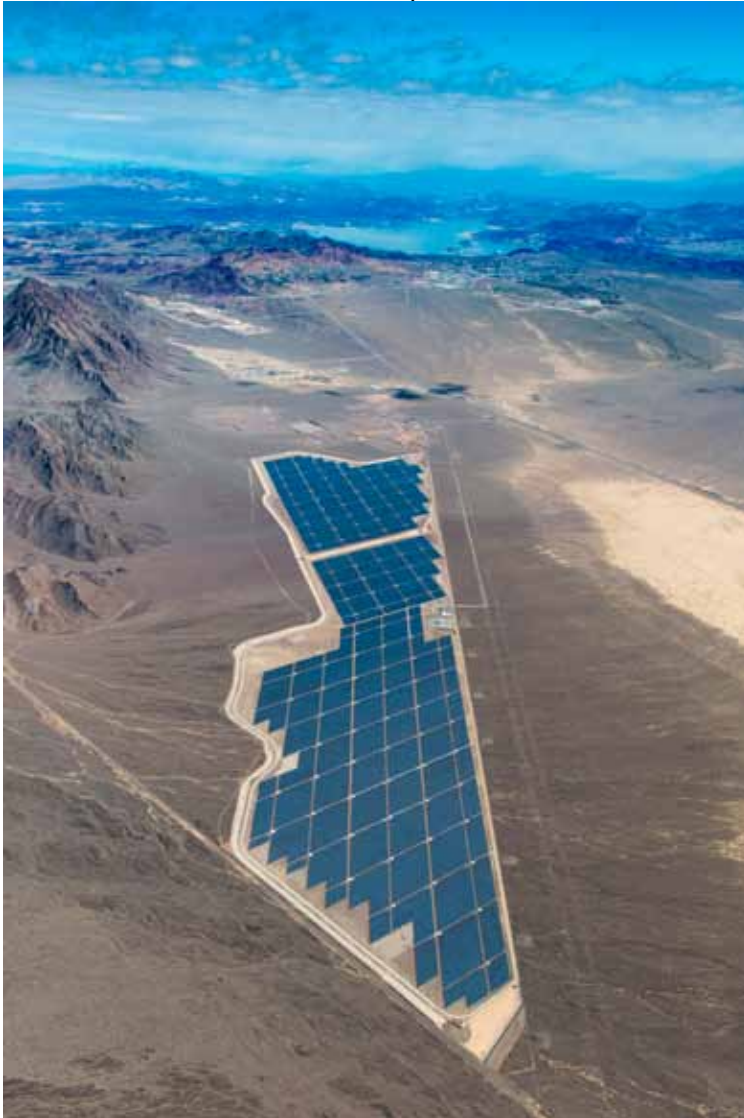
Photo: Copper Mountain 5 (Source: Sempra Energy).
