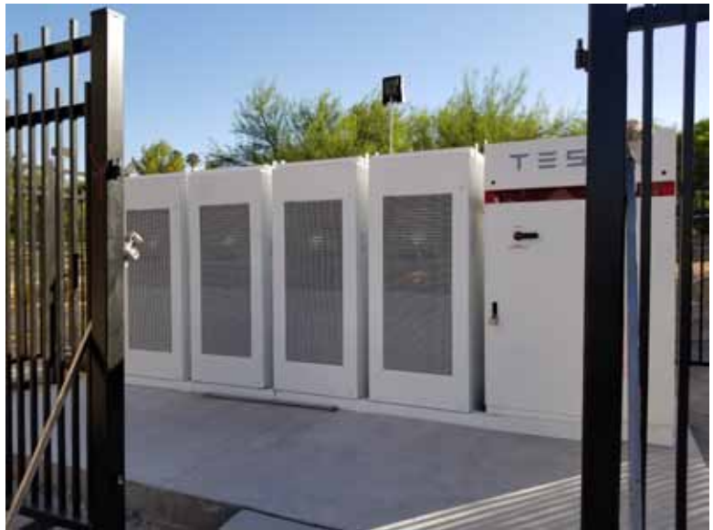
Photo (Above): 210 kW Battery Project at the Grant Sawyer State office building in Las Vegas, NV. (Source: Viridity Energy)
